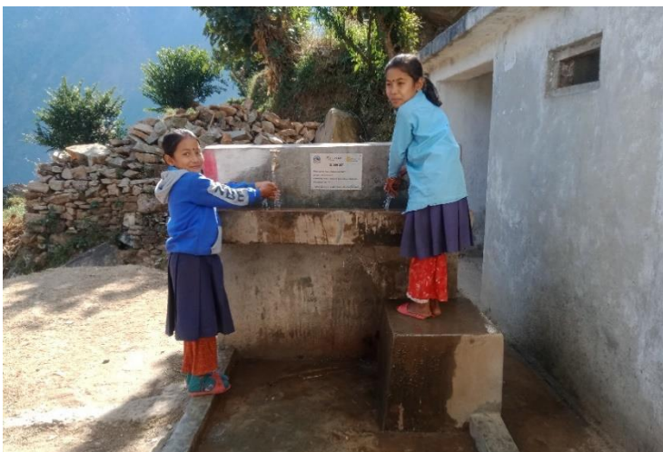
Students using the water tap stands constructed in the school
